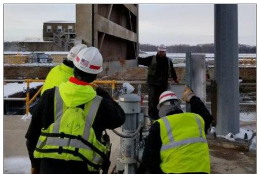
The team preps one of the tainter valve pits in order to remove the tainter valve. The work was performed by the maintenance and repair section as part of the tainter valve rehabilitation at Lock and Dam 4 near Alma, Wisconsin. USACE courtesy photo
